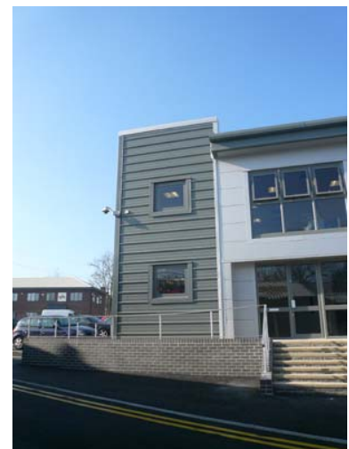
Left Apollo's dedicated entrance to the 2-storey office with the stores to the right
